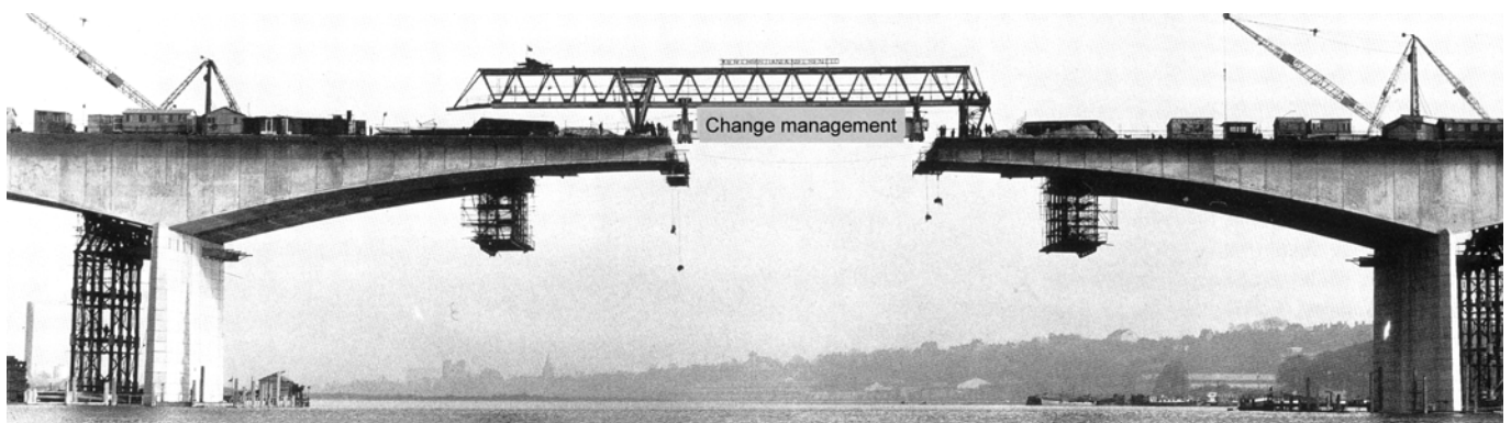
Change management creates the link between the old and the new. Picture taken from "Bridges - 3000 years of defying nature" by David J. Brown.
